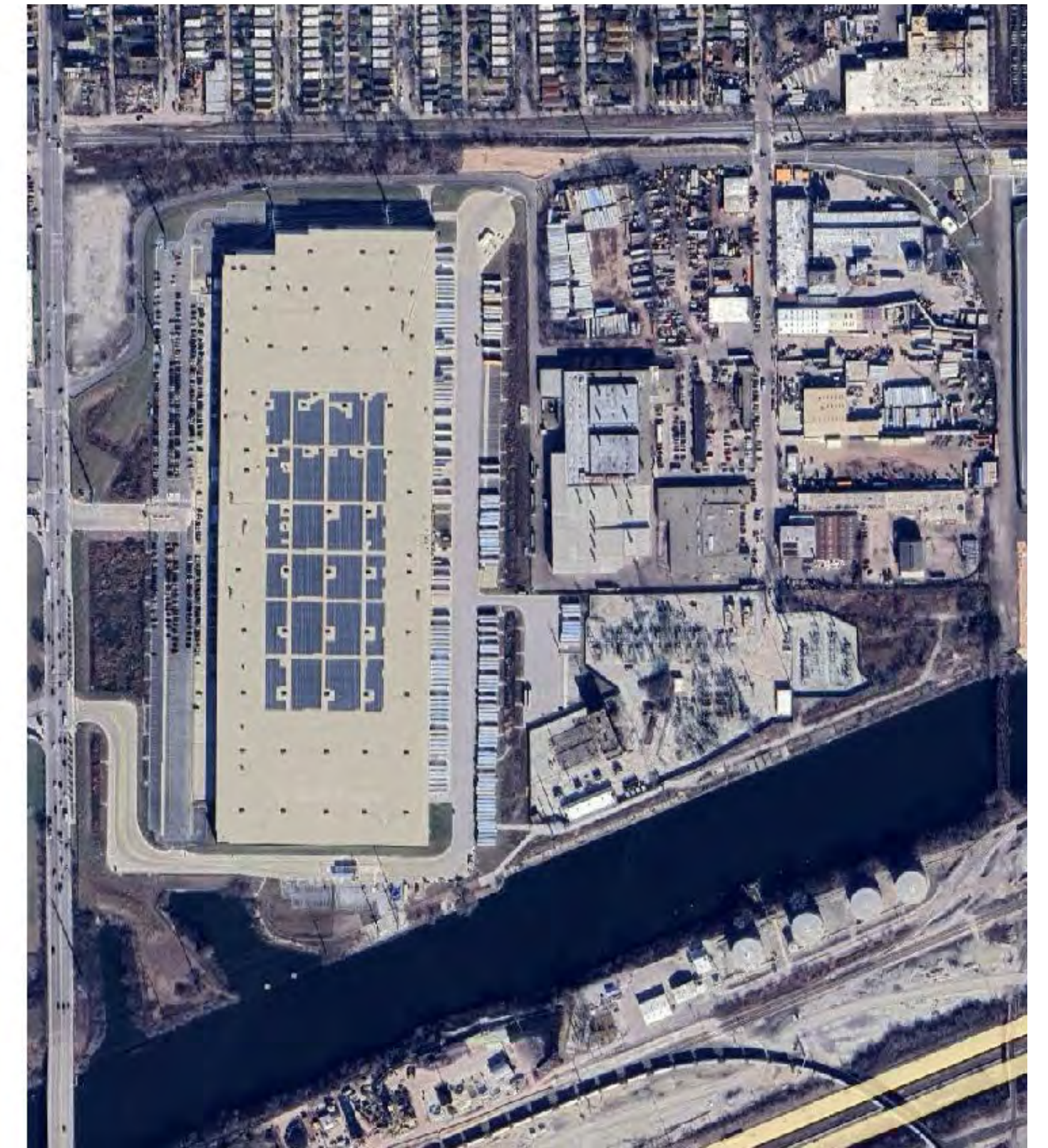
Target Distribution Center, 2024
